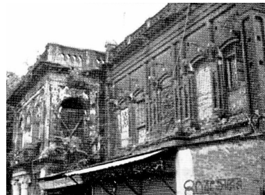
Figure-06: The front view of Building no. 01.
