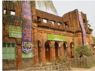
Figure-05: The front view of Building no. 40.
